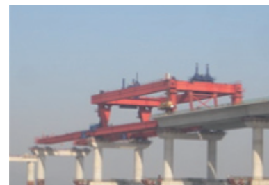
⑫ Launching Girder Self-launching
